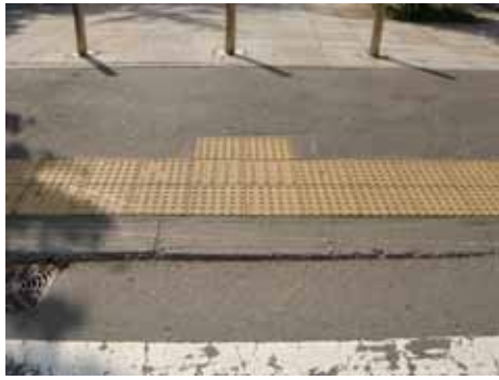
Fig. 55: It is ordinarily best to install two rows of warning blocks before a crosswalk. Where directional blocks are followed by only a single row of warning blocks, as shown here, people with impaired vision may either fail to notice the warning blocks and walk out into the road or inadvertently step over the warning blocks and come to a stop after stepping out into the road. Two rows of warning blocks should be installed as in the improved version. ( Hokkaido, Japan )
