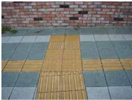
Fig. 53: Here, a single row of directional blocks leads to the wall followed by warning blocks signaling the end of the line. These blocks are unnecessary. As in the improved version, the warning blocks signaling the intersection alone are sufficient. ( Wakayama, Japan )
