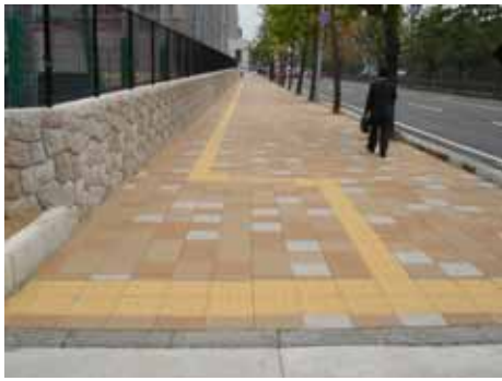
Fig. 50: This is an example of an unnecessary bend in a directional block installation preceding a crosswalk. The directional blocks should simply continue straight ahead as in the improved version. ( Wakayama, Japan )
