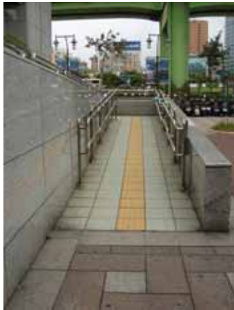
Fig. 32: Tactile Ground Surface Indicators Installed on a Slope (Taipei, Taiwan)
