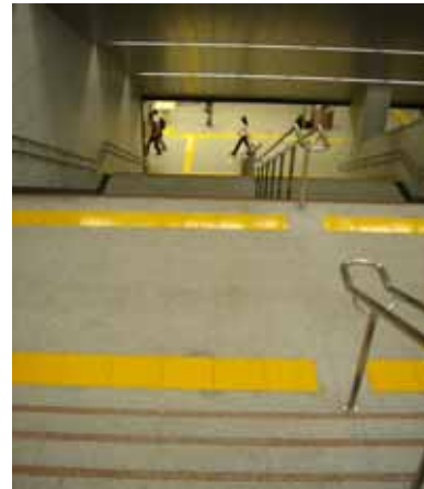
Fig. 75: Warning blocks should be installed across the entire width of the stairway, as shown here. The one-block interruption at the center of the rows of warning blocks is due to the position of the handrail. ( Ibaraki, Japan )
