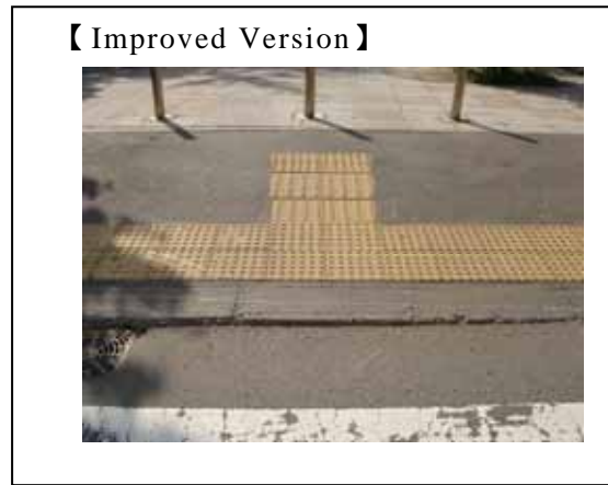
Fig. 55: It is ordinarily best to install two rows of warning blocks before a crosswalk. Where directional blocks are followed by only a single row of warning blocks, as shown here, people with impaired vision may either fail to notice the warning blocks and walk out into the road or inadvertently step over the warning blocks and come to a stop after stepping out into the road. Two rows of warning blocks should be installed as in the improved version. ( Hokkaido, Japan )
