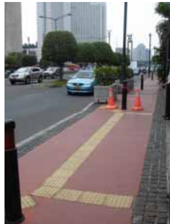
Fig. 23: Tactile Ground Surface Indicators Used to Indicate Parking Lot Entrances (Jakarta, Indonesia)
