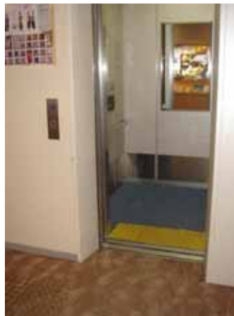
Fig. 86: Warning blocks are sometimes installed inside elevators. People with impaired vision, however, will not lose track of the entrance within the narrow confines of an elevator. Such blocks are an obstacle to wheelchair use and should be removed. ( Ehime, Japan )
