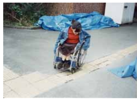
Fig. 97: Broken blocks not only pose a danger to people with impaired vision but are also a major barrier for wheelchair users.
