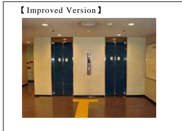
Fig. 85: Tactile ground surface indicators installed in this way create a barrier for wheelchair users. Blocks should instead be installed only before the call buttons as shown in the improved version. ( Osaka, Japan )
