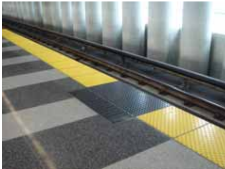
Fig. 18: Tactile Ground Surface Indicators at a Rail Station Platform (San Francisco, USA)
