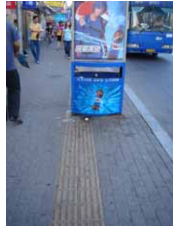
Fig. 103: A bus stop covering a line of directional blocks.
