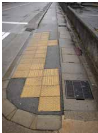
Fig. 55: It is ordinarily best to install two rows of warning blocks before a crosswalk. Where directional blocks are followed by only a single row of warning blocks, as shown here, people with impaired vision may either fail to notice the warning blocks and walk out into the road or inadvertently step over the warning blocks and come to a stop after stepping out into the road. Two rows of warning blocks should be installed as in the improved version. ( Hokkaido, Japan )
