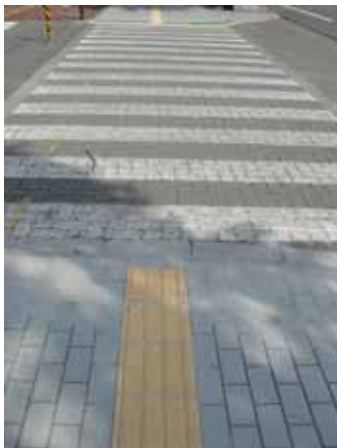
Fig. 54: Situations like this one are extremely dangerous as people with impaired vision, rather than stopping before the crosswalk, will step out into traffic as they search for the continuation of the line of directional blocks. Warning blocks should be installed as in the improved version. ( Hokkaido, Japan )
