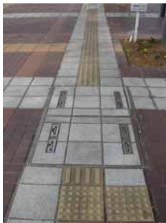
Fig. 34: As in this instance, manhole covers often interrupt the flow of directional blocks, causing people with impaired vision to lose track of which direction they should proceed. ( Tokyo, Japan )
