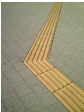
Fig. 41: The angle here is 130^\circ so warning blocks should be installed as in the improved version. ( Kanagawa, Japan )
