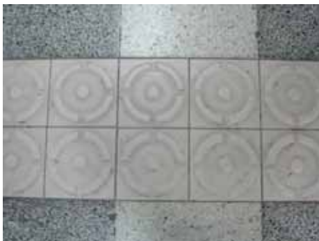
Fig. 19: Blocks Used in Some Seoul Subway Stations (Seoul, Korea)
