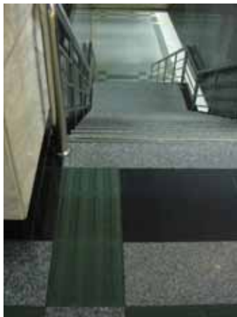
Fig. 69: Here there are no warning blocks at the top of the stairs. Unable to stop, people with impaired vision may fall down the stairs. (Guangzhou, China)
