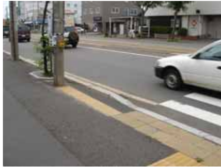
Fig. 60: Many crosswalks are outfitted with pushbutton-operated signals for pedestrians. In this case, a pushbutton accessible to people with disabilities has been installed. Installations of directional blocks leading to such pushbuttons are rarely seen, yet are helpful in enabling people with impaired vision locate the pushbuttons. ( Hokkaido, Japan )
