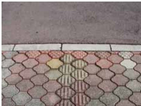
Fig. 49: In this case, the exceptionally small area covered by the warning blocks creates the danger that people with impaired vision will step out into the crosswalk before noticing them. ( Okinawa, Japan )
