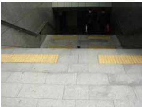
Fig. 68: Here, the line of warning blocks installed at the top of the stairs is truncated. A person with impaired vision arriving at the open gap would fail to come to a stop as there are no warning blocks. There is a real danger of falling down the stairs. The line of warning blocks should be continuous as in the improved version. ( Toyama, Japan )
