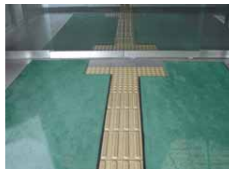
Fig. 105: Rather than cover the Tactile ground surface indicators with the mats, the mats should be shaped as shown to leave the blocks uncovered. ( Hiroshima, Japan )
