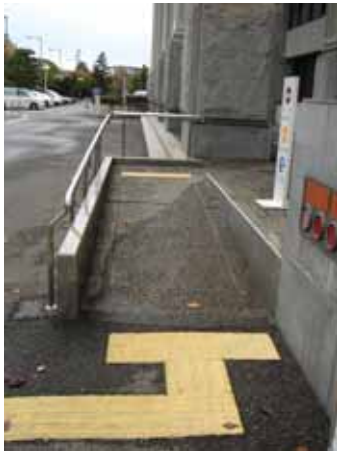
Fig. 83: Blocks are often installed at the beginning and end of slopes, but this creates a barrier for wheelchair users. ( Ehime, Japan )
