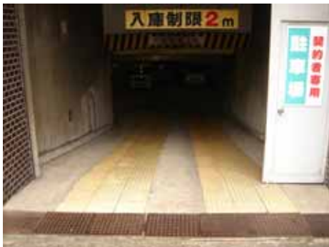
Fig. 107: Tactile ground surface indicators are sometimes used, as shown here, to create a non-slip surface at the entrances to underground parking areas. (Wakayama, Japan)
