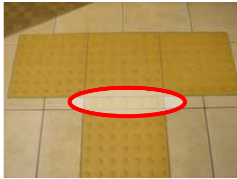
Fig. 46: A directional block of but 5cm width sandwiched between warning blocks, as pictured here, will go unnoticed by people with impaired vision. ( Tokyo, Japan )
