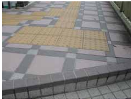
Fig. 72: Here, warning blocks have been installed in a way that is neither adjacent nor parallel to the edge of the stairs. ( Nagasahi, Japan )
