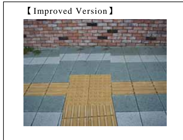
Fig. 53: Here, a single row of directional blocks leads to the wall followed by warning blocks signaling the end of the line. These blocks are unnecessary. As in the improved version, the warning blocks signaling the intersection alone are sufficient. ( Wakayama, Japan )
