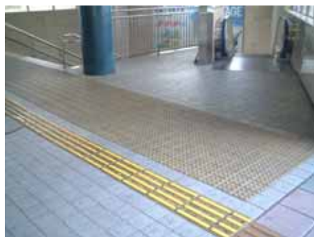
Fig. 73: Situations like this one where there are many warning blocks installed make it difficult for people with impaired vision to determine what is in their surroundings. There is a danger that they could fall down a stairs or an escalator while searching about. Double rows of warning blocks are sufficient before both stairs and escalators. ( Toyama, Japan )
