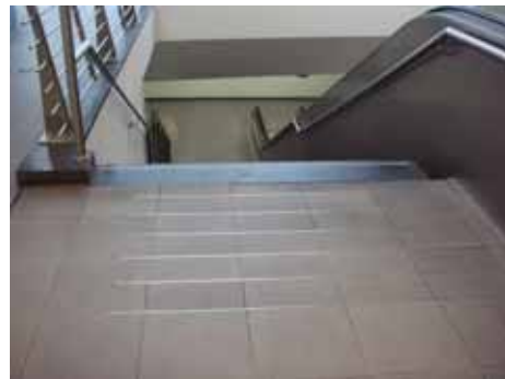
Fig. 11: Embedded Metal Bars Marking the Top of a Stairway (Brussels, Belgium)
