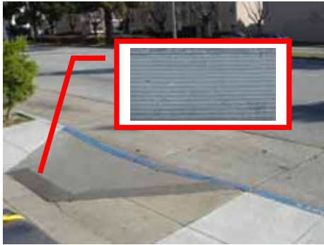
Fig.16: Shallow Grooves Cut into the Pavement before a Crosswalk (San Francisco, USA)
