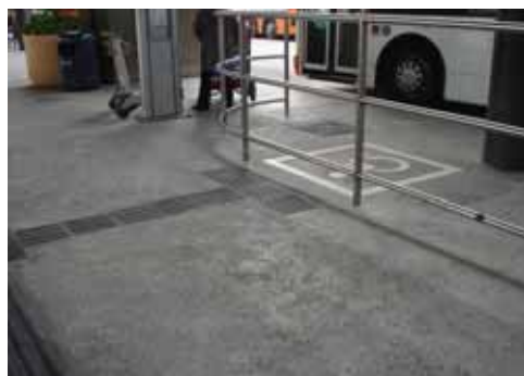
Fig. 93: Here it is impossible to follow the Tactile ground surface indicators to the bus stop due to fencing that was installed later. (Hong Kong)
