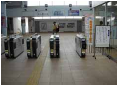
Fig. 87: Here, the wicket where Tactile ground surface indicators are installed is correctly separate from the wider wicket for wheelchair users. ( Ibaraki, Japan )
