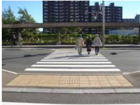
Fig. 63: Wide medians like this one can cause people with impaired vision to mistakenly think they have crossed the road, so blocks need to be installed in accordance with the proper rules. Blocks installed over the entire surface, as is the case here, are cause for user confusion. Accordingly, installations should be consistent in using double rows of warning blocks at either end of the crosswalk and single rows of warning blocks on either side of the median. ( Hokkaido, Japan )
