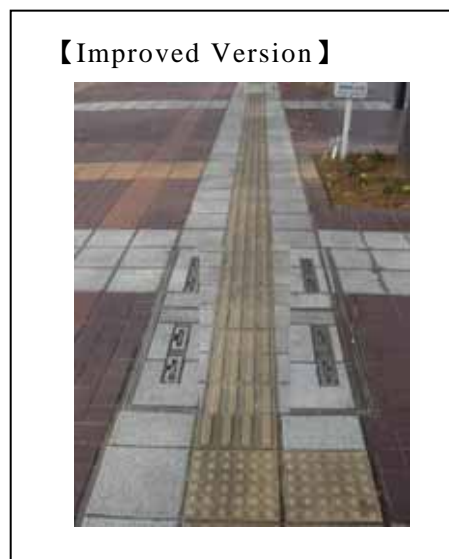
Fig. 34: As in this instance, manhole covers often interrupt the flow of directional blocks, causing people with impaired vision to lose track of which direction they should proceed. ( Tokyo, Japan )
