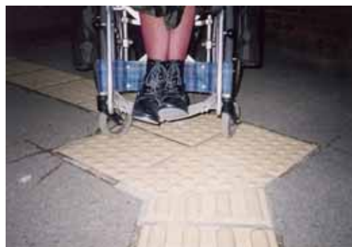
Fig. 80: As depicted here, the protrusions on Tactile ground surface indicators can cause wheelchair wheels to change direction, making it difficult to move forward.
