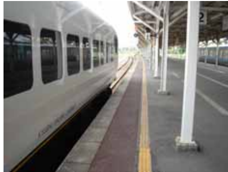
Fig. 77: Here the warning blocks measure only 15cm wide. There is the risk that people with impaired vision may inadvertently step over the blocks and fall onto the tracks. Warning blocks measuring 30cm square should be used on platforms. ( Nagasaki, Japan )
