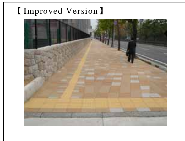
Fig. 50: This is an example of an unnecessary bend in a directional block installation preceding a crosswalk. The directional blocks should simply continue straight ahead as in the improved version. ( Wakayama, Japan )
