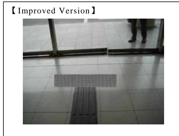
Fig. 79: Here a line of directional blocks ends without warning blocks before a door. Because people with impaired vision will continue toward the door without stopping, there is the risk that they could hit their head on the edge of the door should it happen to be open. Warning blocks should be installed as in the improved version. ( Osaka, Japan )
