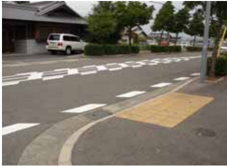
Fig. 91: Here the Tactile ground surface indicators have been left behind after the crosswalk that they marked was eliminated. There is a danger that people with impaired vision will mistakenly believe there to be a crosswalk and attempt to cross the road. ( Osaka, Japan )
