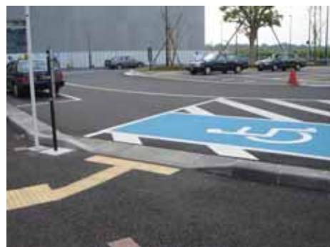
Fig. 90: Because disabled parking spaces are established primarily for wheelchair users, Tactile ground surface indicators should not be installed. ( Chiba, Japan )
