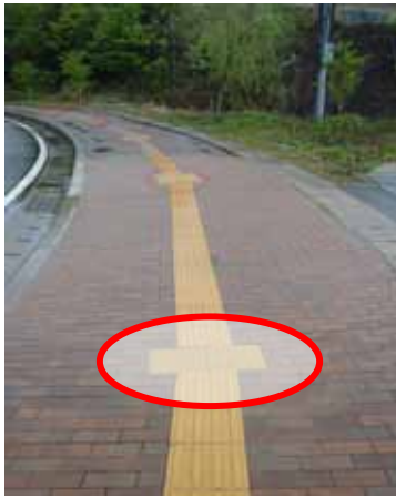
Fig. 42: Installing warning blocks at shallow bends such as these means people with impaired vision must frequently come to a stop. ( Nagasaki, Japan )
