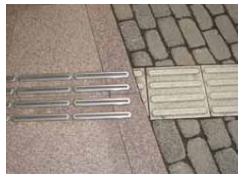
Fig. 39: Situations such as this one, where both shape and materials differ, make it difficult for people with impaired vision to walk and are also unattractive. ( Tokyo, Japan )
