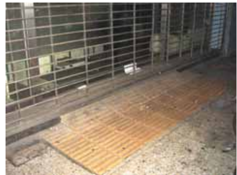
Fig. 108: Here, at the entrance to a store, Tactile ground surface indicators are used to create a non-slip surface as in Fig. 107. (Taipei, Taiwan)
