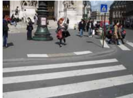
Fig. 100: This photograph, taken before the Paris Opera House, shows the unattractive result of repair using a different type of blocks than those originally used. (Paris, France)
