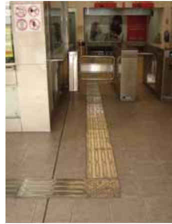
Fig. 88: In fact, there are many cases where Tactile ground surface indicators are installed at the wider, manned wickets. (Kuala Lumpur, Malaysia)
