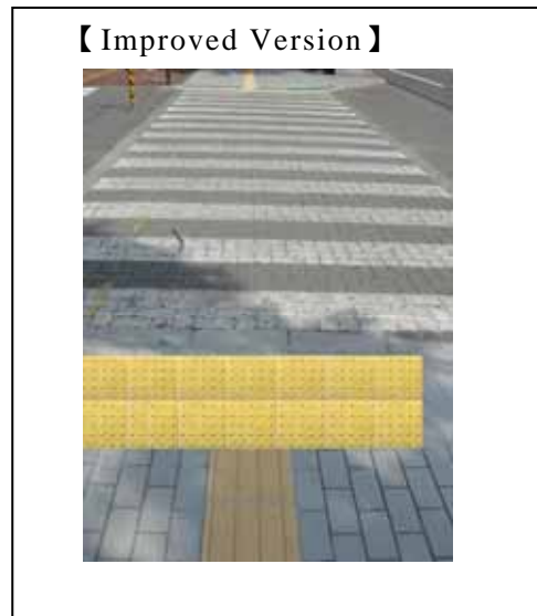
Fig. 54: Situations like this one are extremely dangerous as people with impaired vision, rather than stopping before the crosswalk, will step out into traffic as they search for the continuation of the line of directional blocks. Warning blocks should be installed as in the improved version. ( Hokkaido, Japan )
