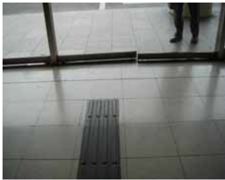
Fig. 79: Here a line of directional blocks ends without warning blocks before a door. Because people with impaired vision will continue toward the door without stopping, there is the risk that they could hit their head on the edge of the door should it happen to be open. Warning blocks should be installed as in the improved version. ( Osaka, Japan )
