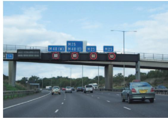
**Figure 6. Example of lane-based variable speed limits (U.K.)**
