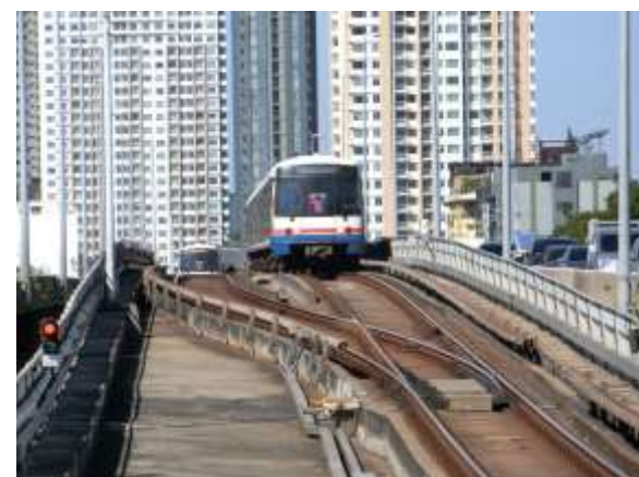
高架通勤鉄道 Elevated Railways (BTS, Bangkok)
