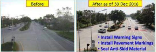
Figure 8-8 The increase of various safety equipment warning the driver to reduce speed
