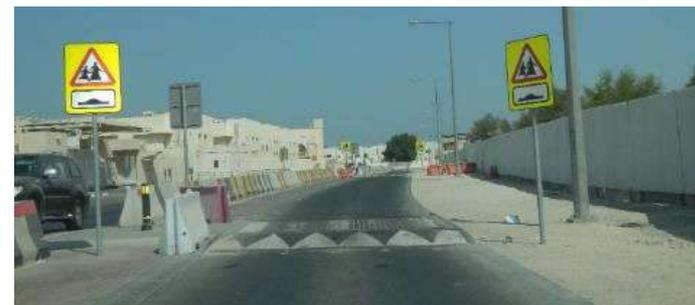
Installation of Speed Suppression Devices at the Locations where Road Hierarchy Changes
