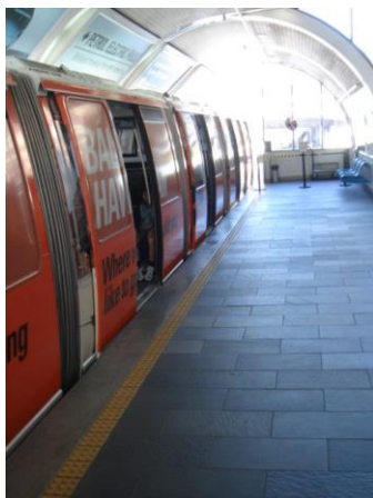
Fig. 25: Use of Narrow (15cm Wide) Warning Blocks (Sydney, Australia)
