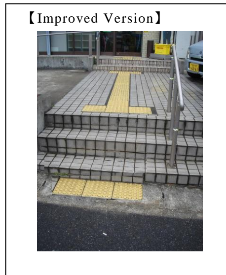
Fig. 70: Warning blocks should generally be installed at the top of stairways and on the ground or floor following the final step. Here, the warning blocks at the bottom of the stairs have been installed not on the ground level but on the final step. People with impaired vision coming down the stairs will sense the warning blocks and determine that they have reached ground level. Because in fact they have an additional step to go, this may lead to accidents such as falls or twisted ankles. Warning blocks should be repositioned as in the improved version. (Aichi, Japan)
