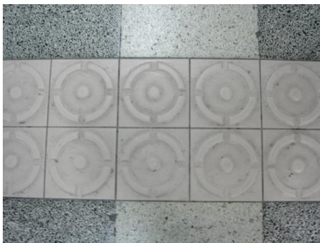
Fig. 19: Blocks Used in Some Seoul Subway Stations (Seoul, Korea)
