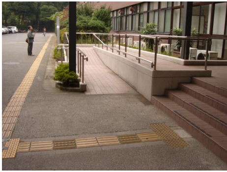
Fig. 81: As shown here, directing people with impaired vision to use the stairs instead of installing Tactile ground surface indicators on the slope eliminates the problem of inconvenience for wheelchair users. (Tokyo, Japan)
