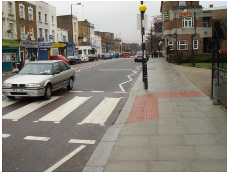
Fig. 3: L-Shaped Tactile ground surface indicator Installation (London, UK)
