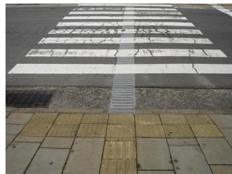
Fig. 59: An example of a crosswalk with escort zone.
