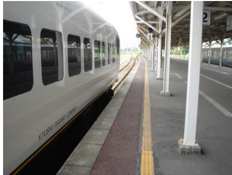
Fig. 77: Here the warning blocks measure only 15cm wide. There is the risk that people with impaired vision may inadvertently step over the blocks and fall onto the tracks. Warning blocks measuring 30cm square should be used on platforms. (Nagasaki, Japan)
