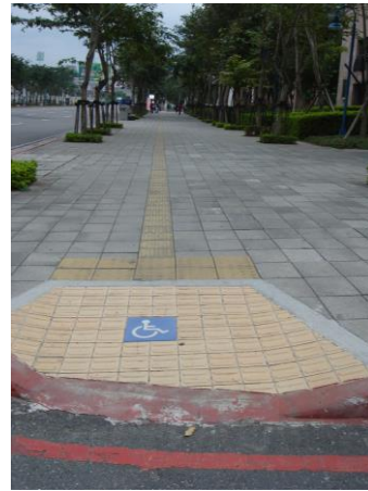
Fig. 21: Blocks Installed Across the Sloped Area before a Crosswalk (Taipei, Taiwan)
