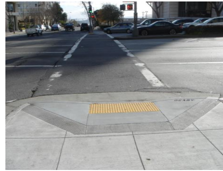
Fig. 17: Tactile Ground Surface Indicators before a Crosswalk (San Francisco, USA)
