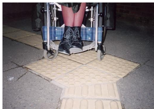
Fig. 80: As depicted here, the protrusions on Tactile ground surface indicators can cause wheelchair wheels to change direction, making it difficult to move forward.
