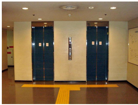
Fig. 85: Tactile ground surface indicators installed in this way create a barrier for wheelchair users. Blocks should instead be installed only before the call buttons as shown in the improved version. (Osaka, Japan)
