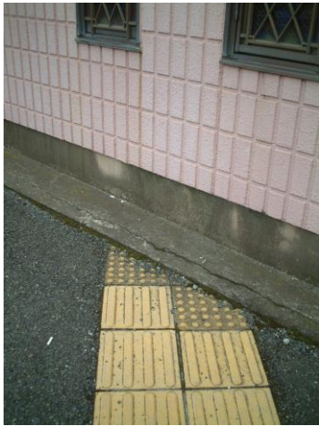
Fig. 48: Because of the small area covered by the warning blocks installed before the wall, people with impaired vision will run into the wall before noticing the warning blocks. (Kanagawa, Japan)
