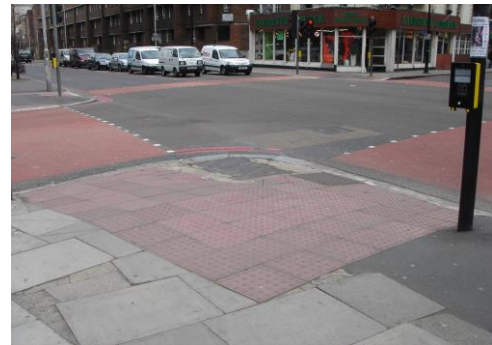
Fig. 62: Covering the sidewalk with blocks as in this example makes it impossible for users to determine where the crosswalks are or which direction to proceed. (London, UK)
