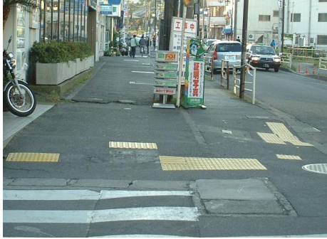
Fig. 94: Because the Tactile ground surface indicators have peeled away before the crosswalk, people with impaired vision may not recognize that there is a crosswalk and step out into the road. (Kanagawa, Japan)
