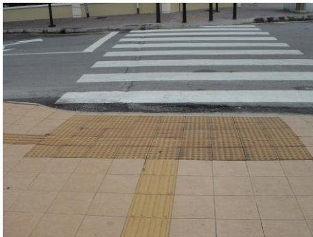
Fig. 61: Examples of numerous Tactile ground surface indicators installed before crosswalks, which can cause people with impaired vision to lose their way, are often seen overseas as well as in Japan. (Kuala Lumpur, Malaysia)
