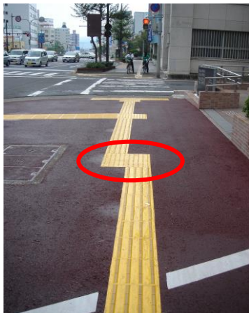
Fig. 51: Here, warning blocks have been installed where the row of directional blocks was shifted over to the left by the width of one block (30cm) before a crosswalk to align the directional blocks with the center of the crosswalk. As long as the directional blocks leading to a crosswalk are not too close to the crosswalk's edge, there is no need to install warning blocks and alter the course of the directional blocks in this way. (Hokkaido, Japan)
