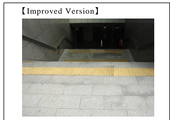
Fig. 68: Here, the line of warning blocks installed at the top of the stairs is truncated. A person with impaired vision arriving at the open gap would fail to come to a stop as there are no warning blocks. There is a real danger of falling down the stairs. The line of warning blocks should be continuous as in the improved version. (Toyama, Japan)
