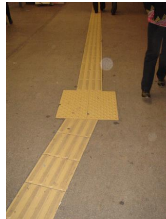
Fig. 31: Installation of Warning Blocks Where They are Unnecessary (Hong Kong)
