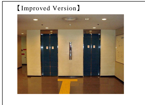
Fig. 85: Tactile ground surface indicators installed in this way create a barrier for wheelchair users. Blocks should instead be installed only before the call buttons as shown in the improved version. (Osaka, Japan)
