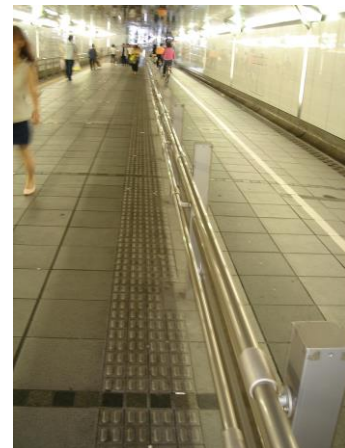
Fig. 52: Directional blocks should not be installed at the edge of walkways because some people with impaired vision, rather than walking directly on top of Tactile ground surface indicators, walk to the side while sensing the texture of the blocks with their canes. This is why it is necessary to leave 30cm open on either side of the directional blocks. Here, the guardrail immediately adjacent to the directional blocks is likely to be an impediment to walking. (Ciba, Japan)
