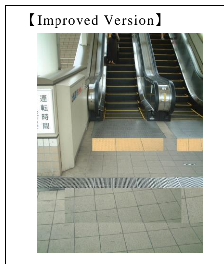
Fig. 76: Here the warning blocks are located too far from the entrance to the escalator, and should instead be installed as in the improved version. (Tokyo, Japan)
