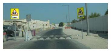
Installation of Speed Suppression Devices at the Locations where Road Hierarchy Changes
