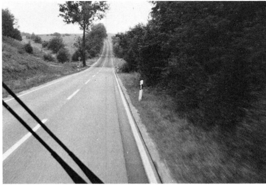
Fig. 12 道路両端に描いた白線 White lines painted on both edges of the road
