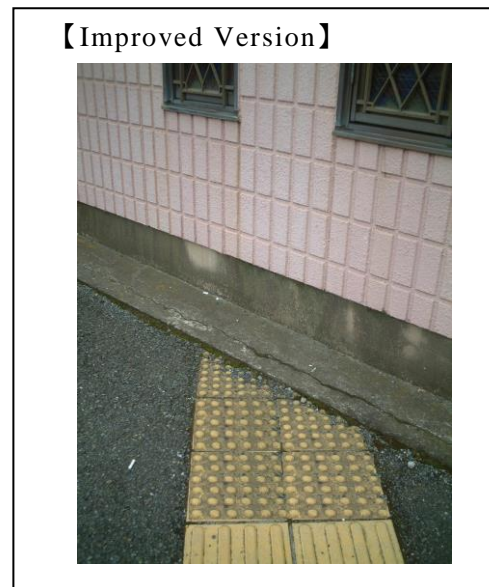
Fig. 48: Because of the small area covered by the warning blocks installed before the wall, people with impaired vision will run into the wall before noticing the warning blocks. (Kanagawa, Japan)
