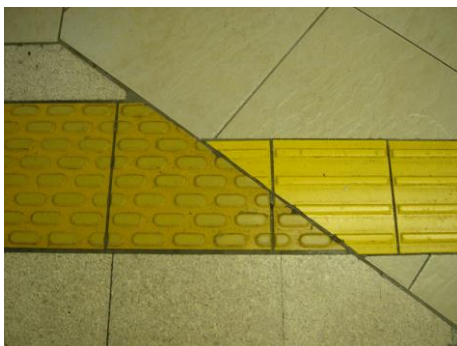
Fig. 38: The situation depicted here is the result of different organizations having jurisdiction over the areas to the left and the right. Both types of blocks are directional blocks but the ones on the left with raised ovals can easily be mistaken for warning blocks with raised dots. The likelihood of misreading the blocks is particularly high when walking from the right to the left. (Tokyo, Japan)
