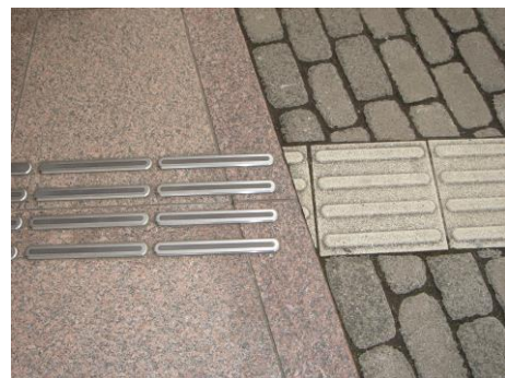
Fig. 39: Situations such as this one, where both shape and materials differ, make it difficult for people with impaired vision to walk and are also unattractive. (Tokyo, Japan)
