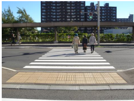
Fig. 63: Wide medians like this one can cause people with impaired vision to mistakenly think they have crossed the road, so blocks need to be installed in accordance with the proper rules. Blocks installed over the entire surface, as is the case here, are cause for user confusion. Accordingly, installations should be consistent in using double rows of warning blocks at either end of the crosswalk and single rows of warning blocks on either side of the median. (Hokkaido, Japan)
