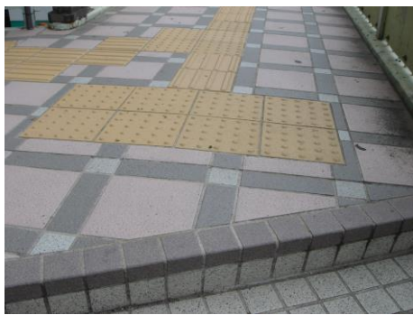
Fig. 72: Here, warning blocks have been installed in a way that is neither adjacent nor parallel to the edge of the stairs. (Nagasaki, Japan)
