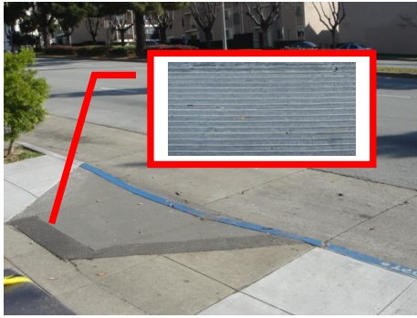
Fig.16: Shallow Grooves Cut into the Pavement before a Crosswalk (San Francisco, USA)
