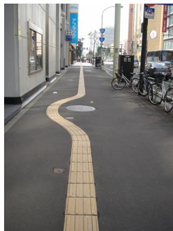
Fig. 36: Rerouting directional blocks to avoid the manhole, as in this photograph, not only looks unattractive but creates a winding course that greatly reduces the walking speed of people with impaired vision. (Hokkaido, Japan)
