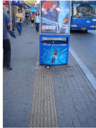
Fig. 103: A bus stop covering a line of directional blocks.
