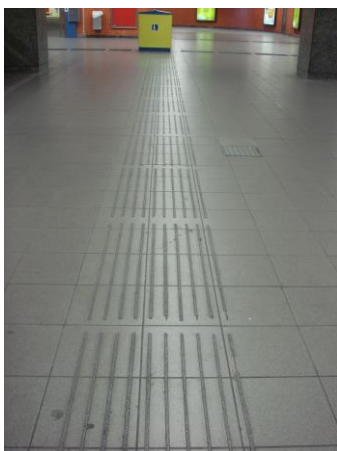
Fig. 12: Embedded Directional Metal Bars (Brussels, Belgium)
