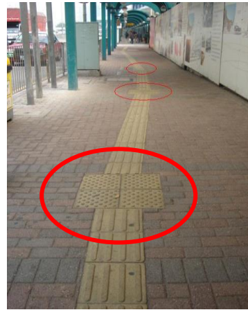
Fig. 43: Many similar examples of the overuse of warning blocks can also be found overseas. (Hong Kong)
