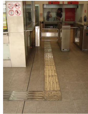
Fig. 88: In fact, there are many cases where Tactile ground surface indicators are installed at the wider, manned wickets. (Kuala Lumpur, Malaysia)
