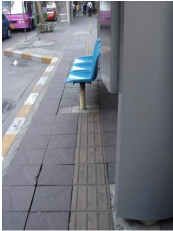
Fig. 102: Benches located above Tactile ground surface indicators at a bus stop in Thailand. (Bangkok, Thailand)
