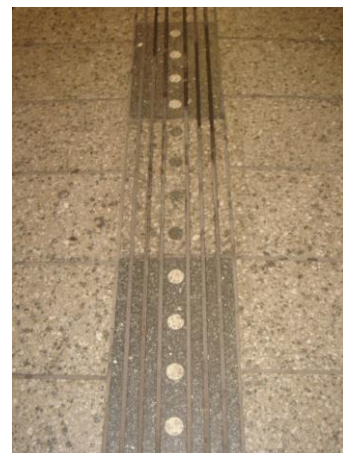
Fig. 15: Grooves Carved into the Pavement (Amsterdam, Netherlands)
