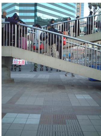
Fig. 28: Pedestrian Bridge Located above Tactile Ground Surface Indicators (Beijing, China)
