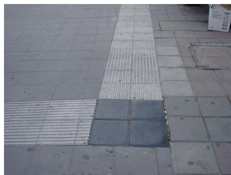
Fig. 13: Rubber Warning Blocks Where Directional Blocks Intersect (Brussels, Belgium)
