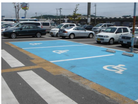
Fig. 89: Here, the extensive installation of Tactile ground surface indicators at disabled parking spaces creates a barrier for wheelchair users. ( Fukushima, Japan)
