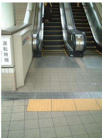
Fig. 76: Here the warning blocks are located too far from the entrance to the escalator, and should instead be installed as in the improved version. (Tokyo, Japan)
