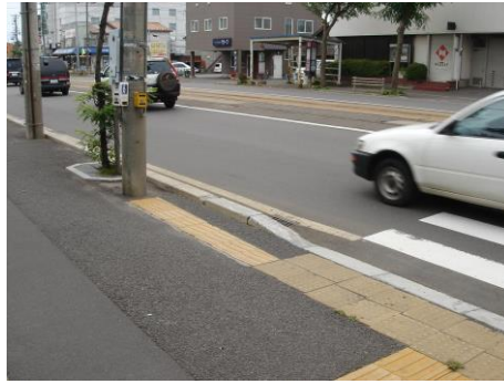
Fig. 60: Many crosswalks are outfitted with pushbutton-operated signals for pedestrians. In this case, a pushbutton accessible to people with disabilities has been installed. Installations of directional blocks leading to such pushbuttons are rarely seen, yet are helpful in enabling people with impaired vision locate the pushbuttons. (Hokkaido, Japan)
