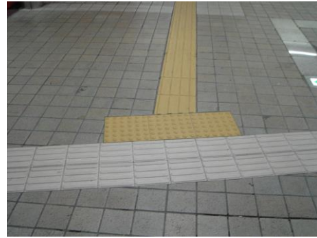
Fig. 67: Warning blocks are sometimes installed in this manner at T-shaped intersections, but such warning blocks will go unnoticed by people with impaired vision who are moving along the path composed of white directional blocks. (Seoul, Korea)
