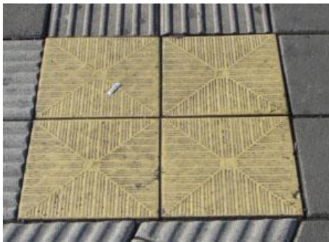
Fig. 14: Netherlands-Style Warning Blocks (Amsterdam, Netherlands)
