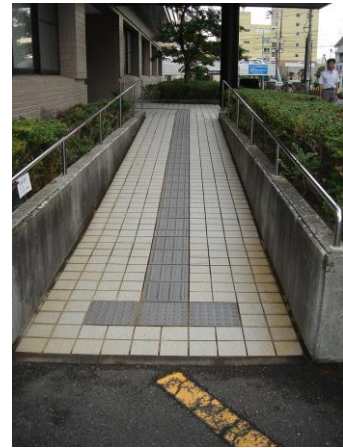
Fig. 82: Installing blocks on a slope as in this example is not appropriate. (Miyazaki, Japan)
