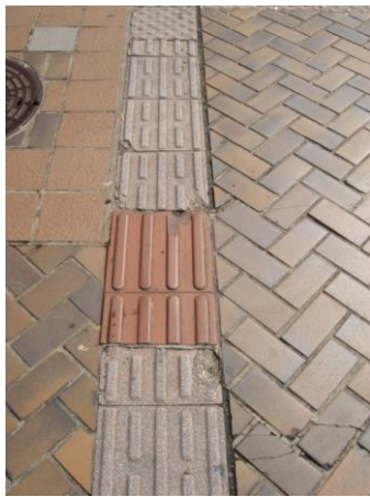
Fig. 99: The use of blocks different than those originally installed is common when Tactile ground surface indicators are repaired. The resulting mix of different specifications and shapes can lead to confusion among people with impaired vision. The loss of visual consistency is also unattractive. (Fukuoka, Japan)
