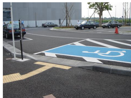
Fig. 90: Because disabled parking spaces are established primarily for wheelchair users, Tactile ground surface indicators should not be installed. ( Chiba, Japan)
