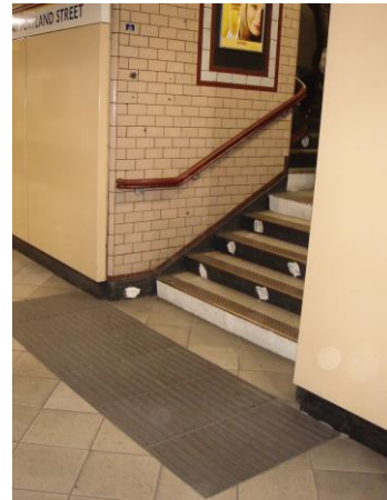
Fig. 4: Blocks with Bars Marking the Bottom of a Stairway (London, UK)
