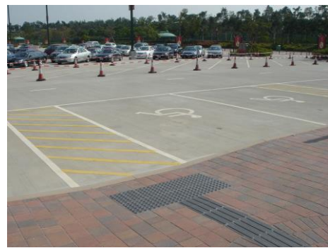
Fig. 33: Tactile Ground Surface Indicators Installed at Disabled Parking Spaces (Hong Kong)
