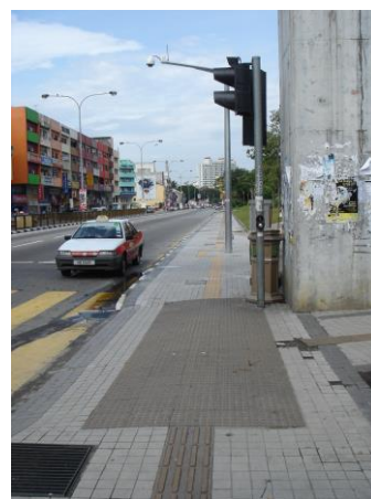
Fig. 29: Installation of an Excessive Number of Blocks (Kuala Lumpur, Malaysia)
