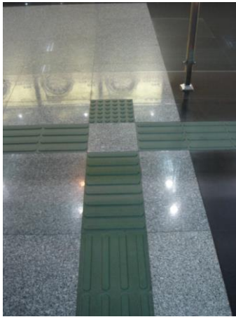
Fig. 20: No Blocks Used Where Directional Blocks Intersect (Guangzhou, China)
